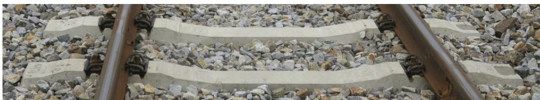
Obr. 4.3.2.14a Pražec B 91T/2 ZK
