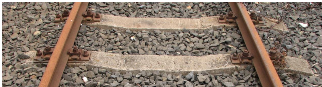
Obr. 4.3.2.2 Pražec SB 3
